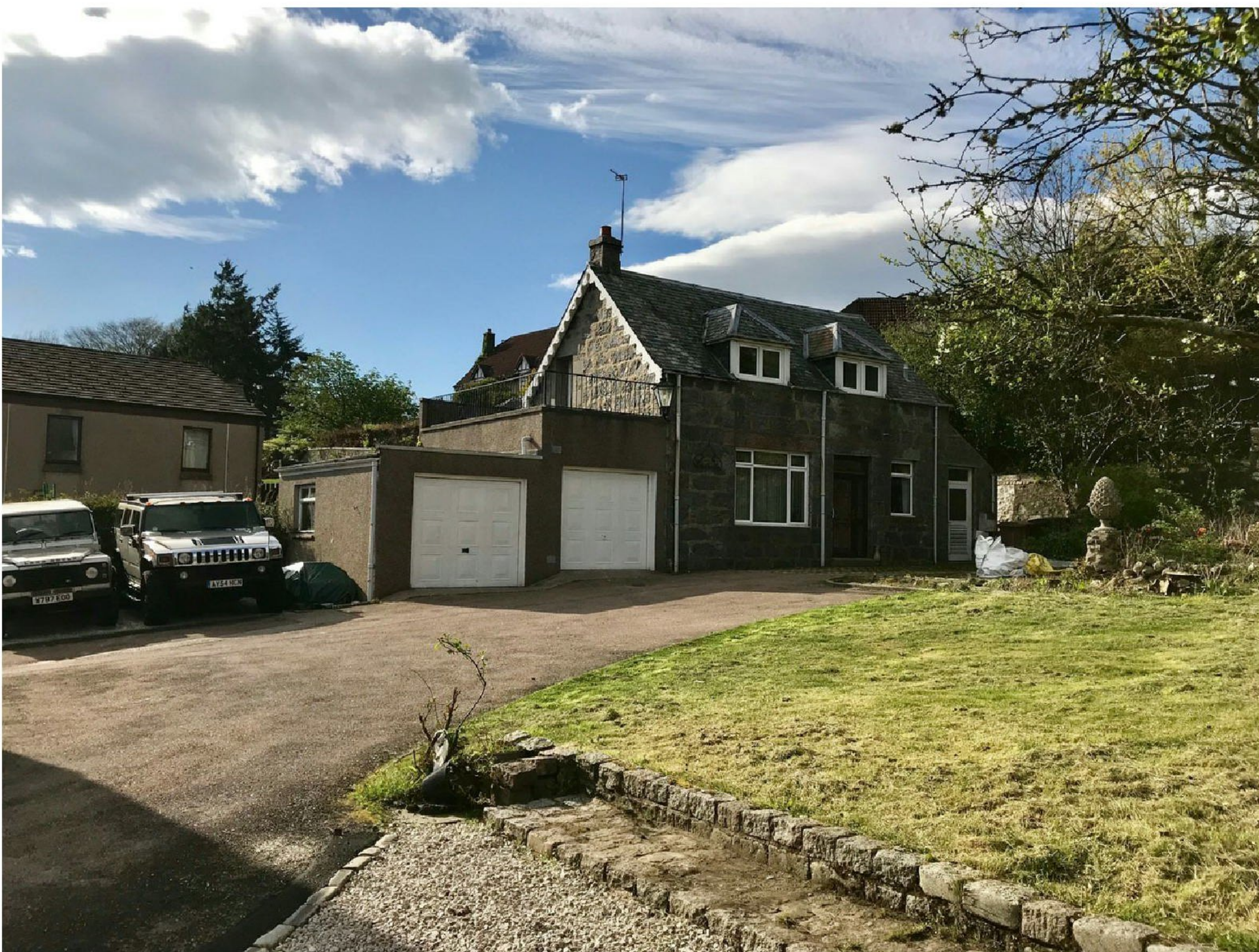
Figure 1 - 108A North Deeside Road
